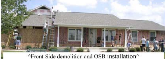
^Front Side demolition and OSB installation^
