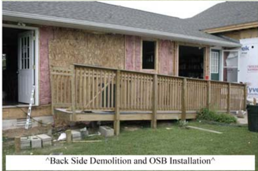
^Back Side Demolition and OSB Installation^
