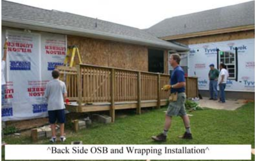
^Back Side OSB and Wrapping Installation^
