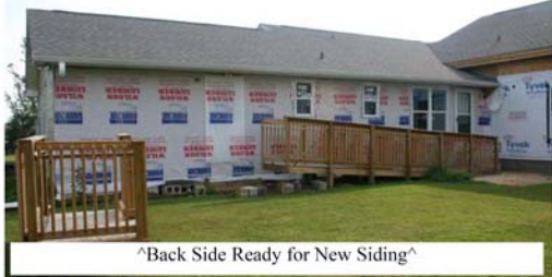
^Back Side Ready for New Siding^
