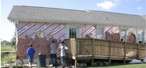
^Back Side Old Siding and Window Removal^
